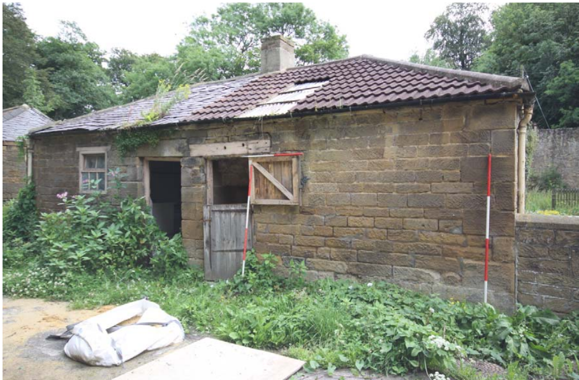
Pl. 10 Buildings 4 and 5, north elevation looking south, (P14 on Fig. 6).
