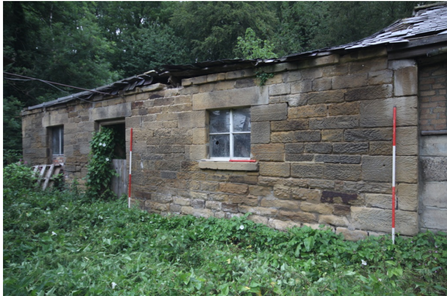
Pl. 12 The western side of Building 6 (P32 on Fig. 7).
