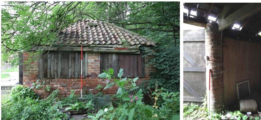
(left) Pl. 6 Building 3 eastern facade looking west. (right) Pl. 7 Detail of rounded bricks on south side on plan (Fig. 5, Pl. 3).
