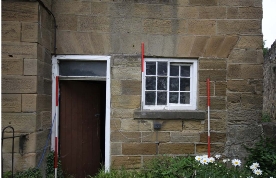
Pl. 13 Western front of Skelton Mill.
