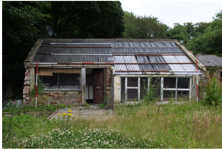
Pl. 4 Image of Building 1 from the west looking east (marked P1 on plan).
